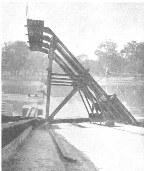
A Trestle being withdrawn from the River at the Mildura Weir.
